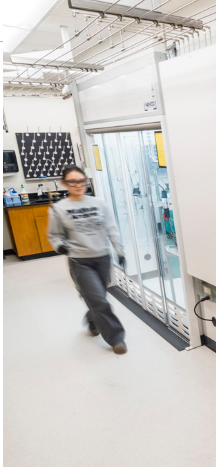
Above: About a mile of tubing lines the ceiling and walls of the Flaherty Lab, carrying dozens of gases.
