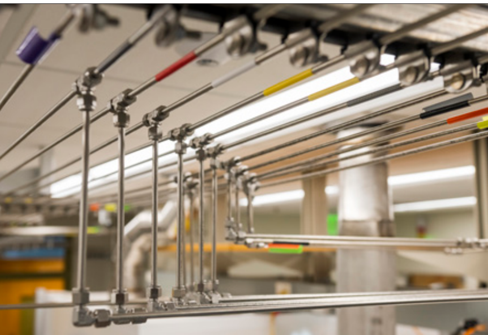
Above: About a mile of tubing lines the ceiling and walls of the Flaherty Lab, carrying dozens of gases.
